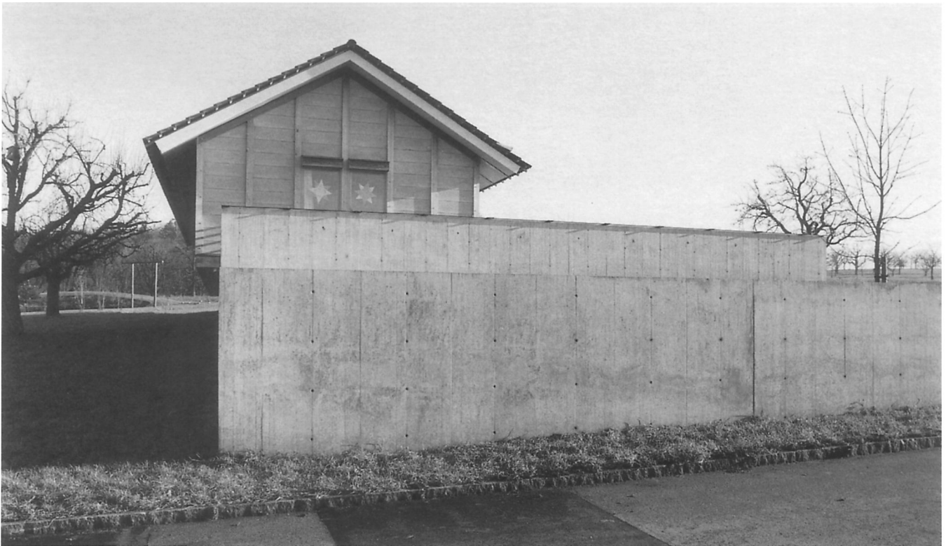
5. View of exterior of courtyard
