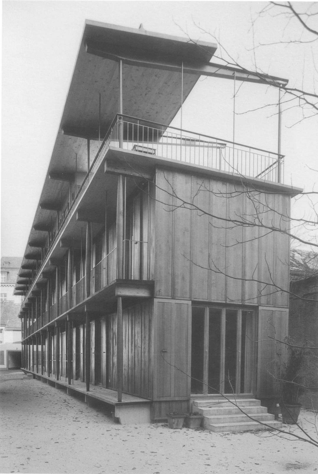
1. View at southwest corner showing roof terrace and door to yard
