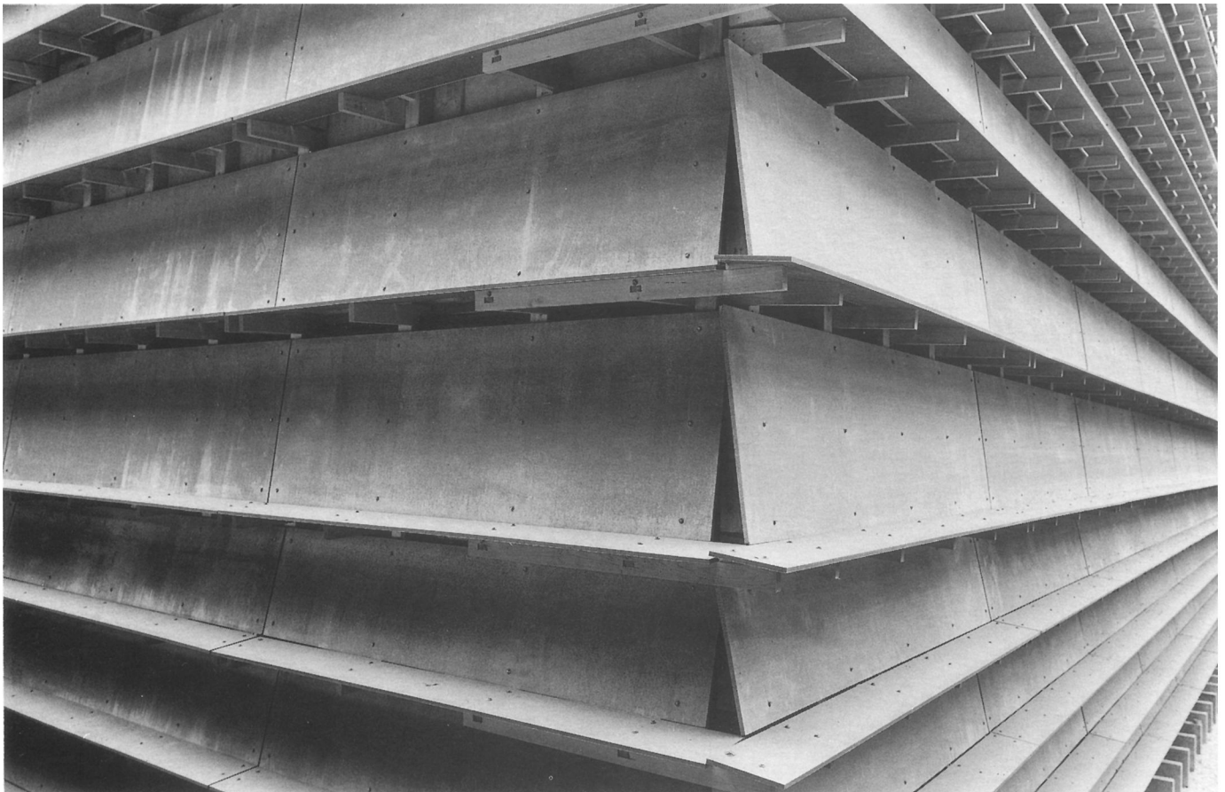
5. View of corner showing cladding system
